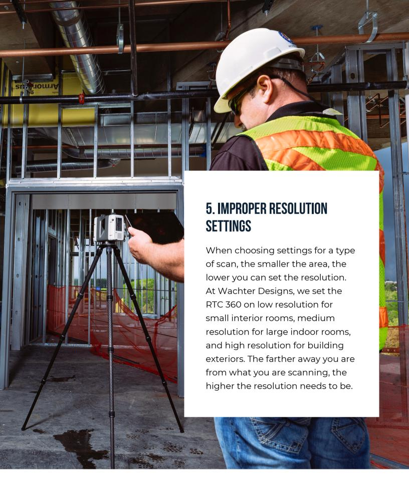
Nothing derails work on improvement projects like inaccurate as-built surveys or drawings. We use cutting-edge LiDAR technology and expert oversight to capture every last detail and keep your projects on track.
